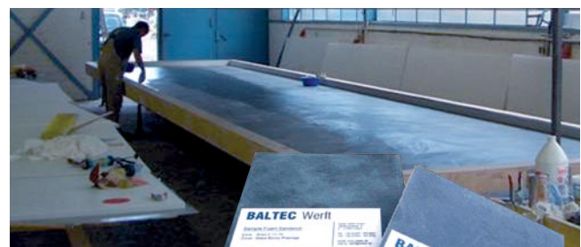
FIGURE 3 The production of large-size GRP (fibreglass-reinforced plastic) sandwich panels occurs in a 12 x 2.4-metre heatable vacuum press.
